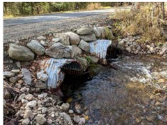
Inlet at Roscoe Road culvert replacement site – Lewis, NY
