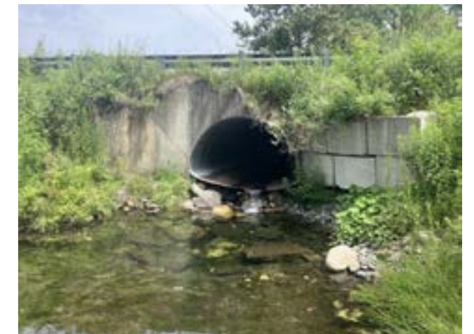
Current structure at Hutchins Farm Road, looking upstream
