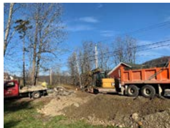
Stormwater project implementation in Wells, VT
