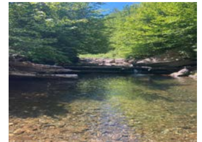
Morses Mill Dam prior to removal. Photo credit Karina Dailey, VNRC
