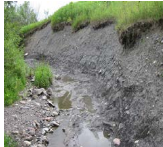
Mass failures along McCabe's Brook (T1.05B) near the Route 7 crossing will be reevaluated as potential sources of sediment and phosphorus requiring mitigation.
