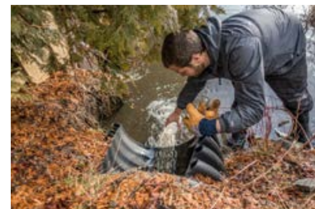
AWI staff collecting a water sample from the stormwater system draining to Mirror Lake.
