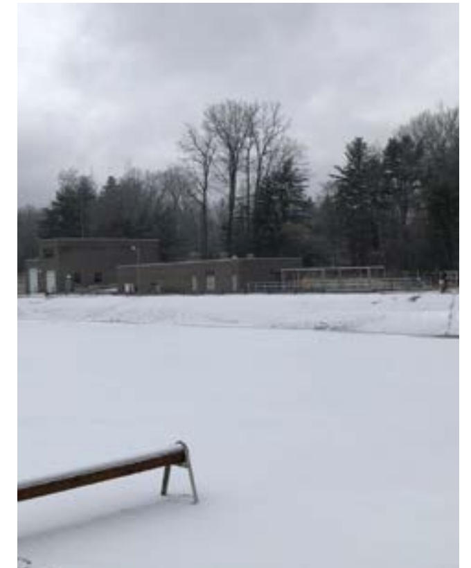
Town of Peru Village Wastewater treatment facility
