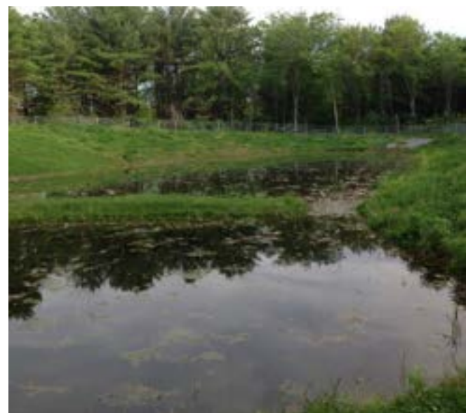
Harrington Village Gravel Wetland constructed in 2014 to treat stormwater in Shelburne, VT is similar to the gravel wetland to be implemented at Burlington Country Club.
