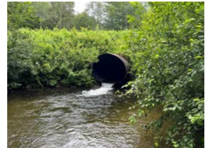
Joes Brook Culvert Outlet, Downstream
