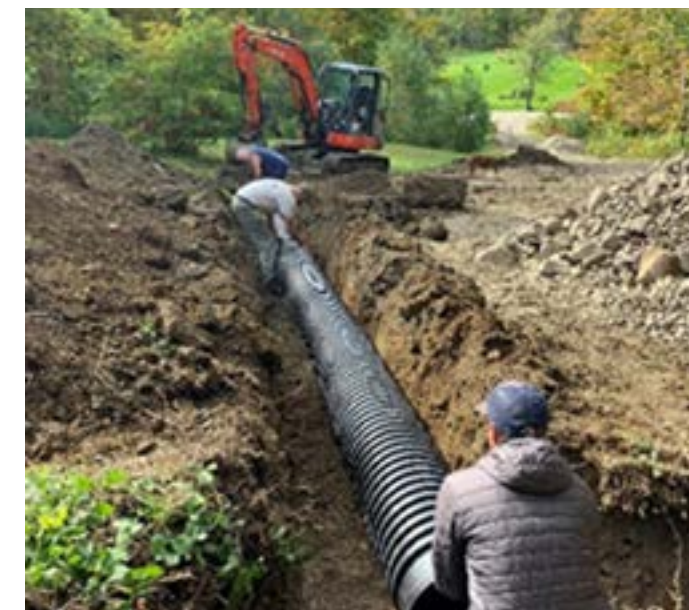
Installation of the cross culvert on one private driveway
